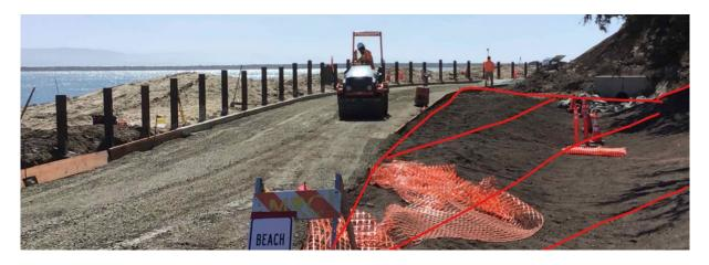
During the last phases of construction it was determined that additional quantities of materials and work would be needed, e.g., additional sand, reinforcement of the headwall footing, installation of erosion control blankets in the bioretention basin to protect bioretention soil from erosion because native vegetation planting had to be postponed due to need to wait for rainy season, installation of additional decomposed granite on the trail between the project area and the parking lot,
