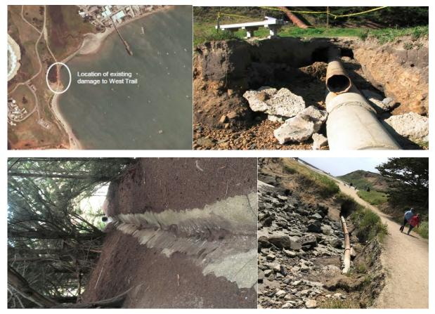
The upper concrete swale located on top of the adjacent bluff was also addressed. The concrete swale channels rainwater from the bluff top to the mouth of a down pipe which was replaced and covered. The upper swale now directs rainwater to a nearby natural marsh wetlands.
